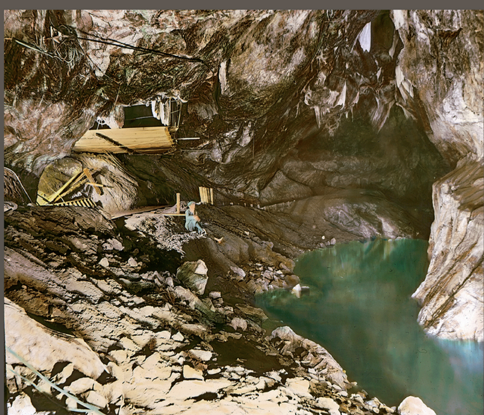
Stavba přístaviště u odbočky k Masarykovu dómu na podzemní plavbě Construction of a dock made near the tunnel leading to the Masaryk's Dome located on water parts of the caves
